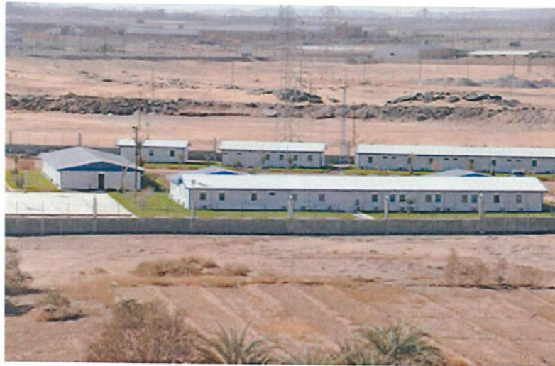
Overview pictures of the plant and camp in Sebha
